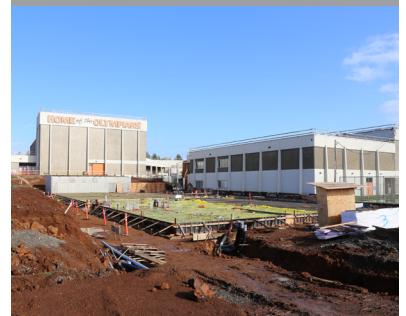
Southwest classroom addition
